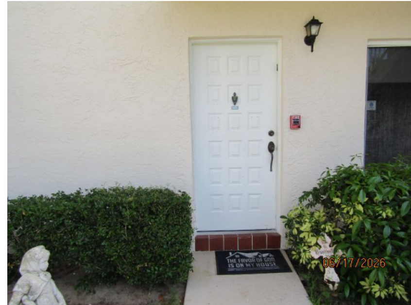
Unprotected Solid Entry Door
