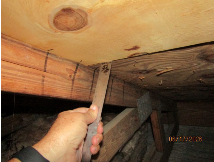
5/8" Deck Thickness Confirmed
