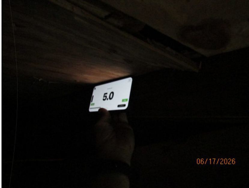
Primary Slope Measurement, Covering 100% of Main Roof
