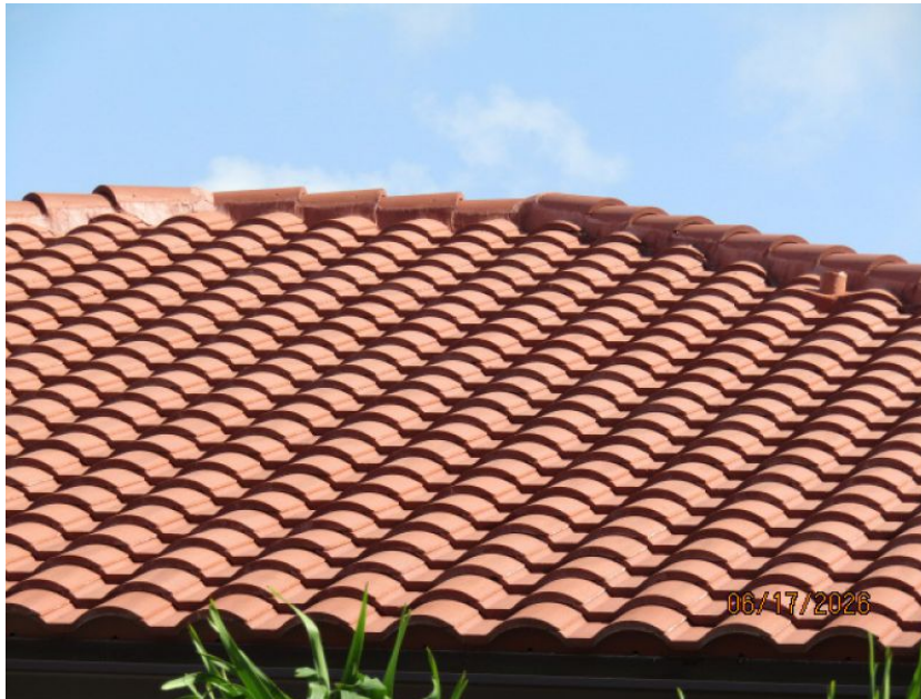
Concrete/Clay Tile Roof Covering
