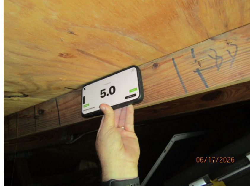
Primary Slope Measurement, Covering 100% of Main Roof
