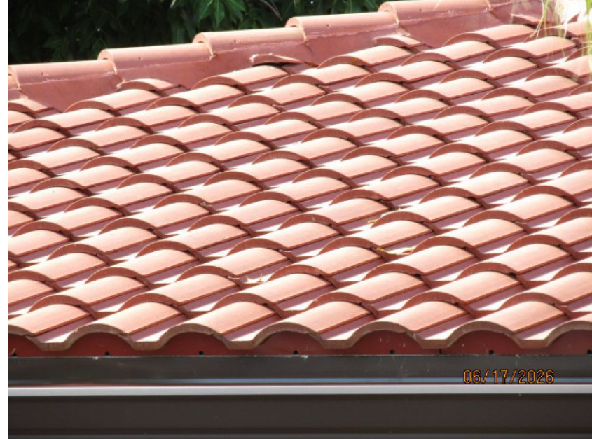
Concrete/Clay Tile Roof Covering
