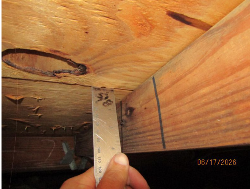
5/8" Deck Thickness Confirmed
