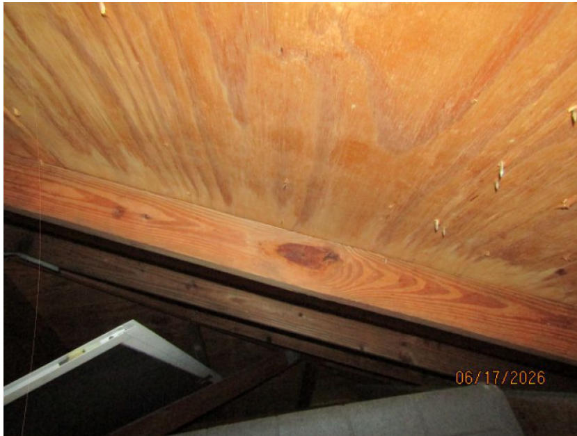
Primary Slope Representative Area, Covering 100% of Main Roof
