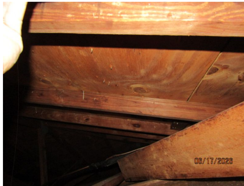
Primary Slope Representative Area, Covering 100% of Main Roof
