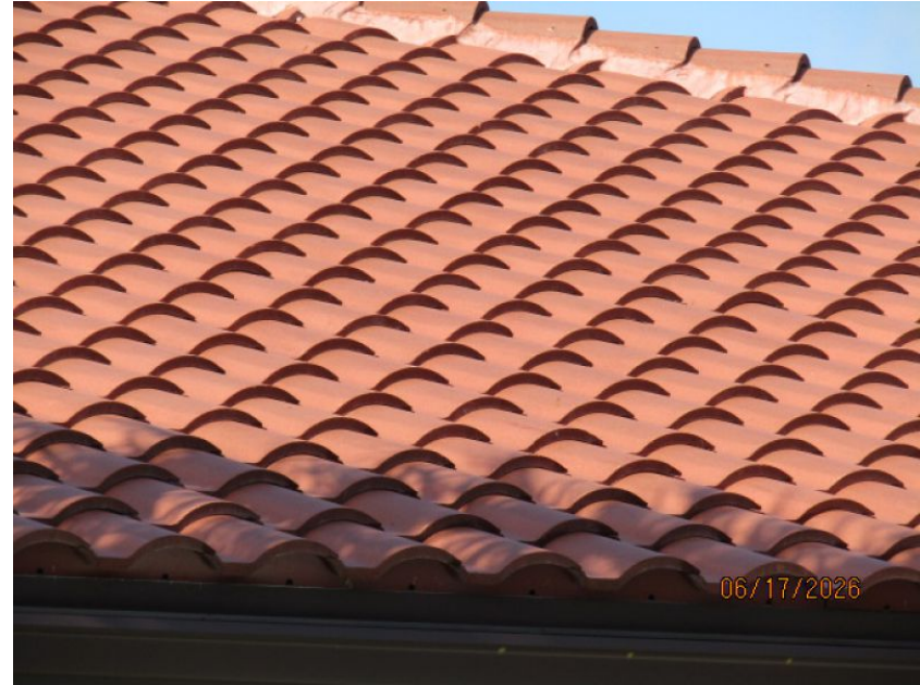
Concrete/Clay Tile Roof Covering
