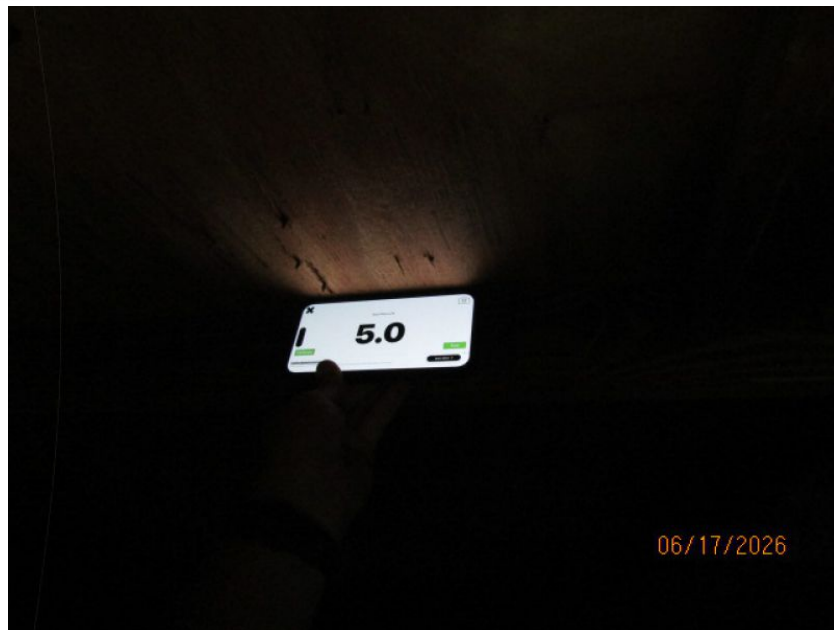
Primary Slope Measurement, Covering 100% of Main Roof
