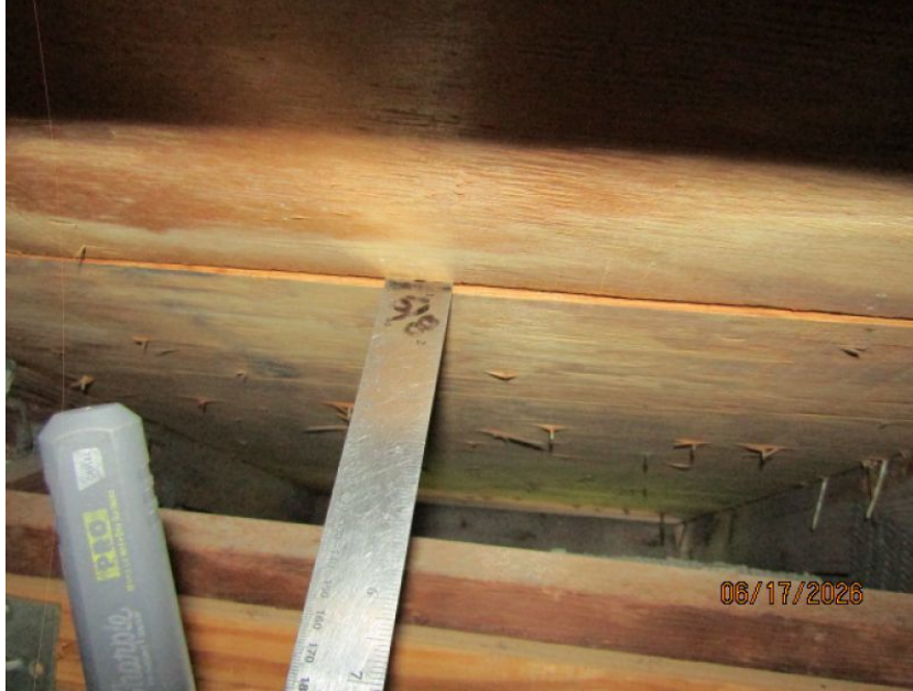
5/8" Deck Thickness Confirmed
