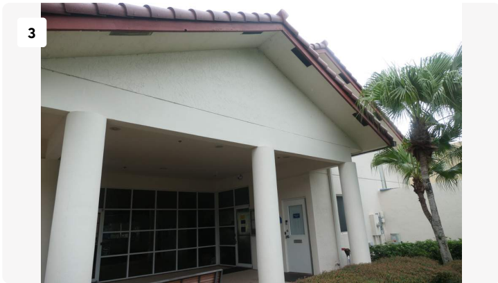
Project: ClubHouse Date: 8/29/2024, 2:12pm Creator: James Stuart
