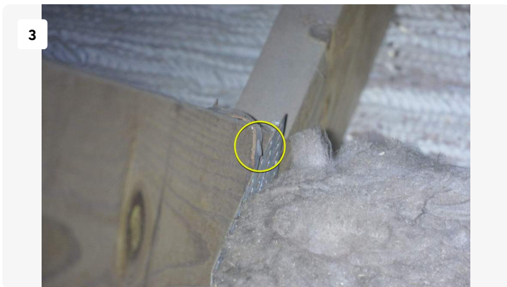
Project: ClubHouse Date: 8/29/2024, 1:30pm Creator: James Stuart
