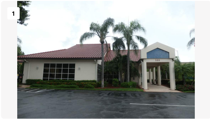
Project: ClubHouse Date: 8/29/2024, 2:06pm Creator: James Stuart
