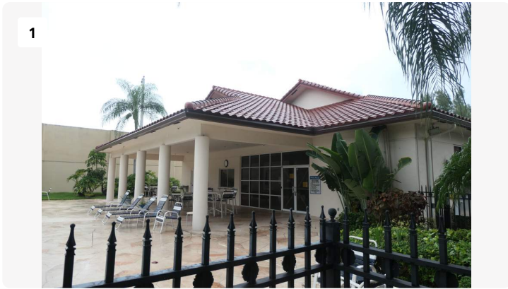
Project: ClubHouse Date: 8/29/2024, 2:07pm Creator: James Stuart
