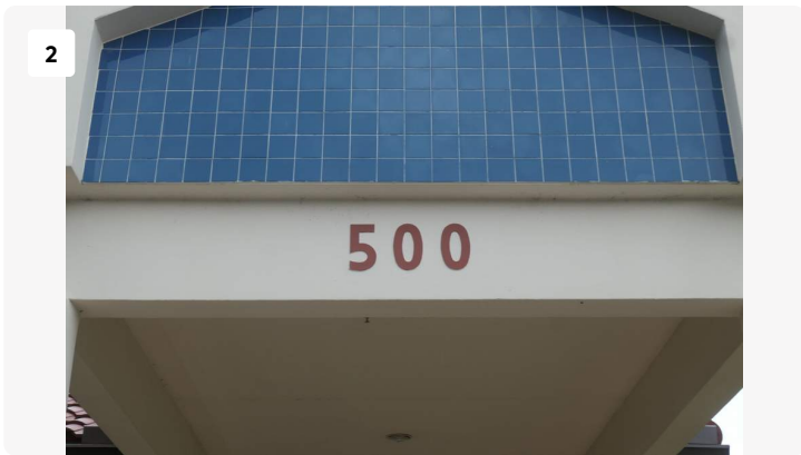
Project: ClubHouse Date: 8/29/2024, 2:06pm Creator: James Stuart
