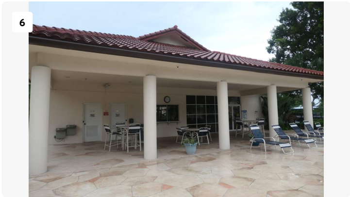
Project: ClubHouse Date: 8/29/2024, 2:09pm Creator: James Stuart
