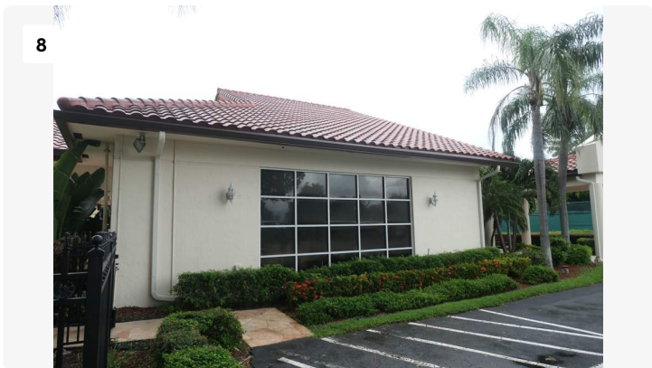
Project: ClubHouse Date: 8/29/2024, 2:07pm Creator: James Stuart
