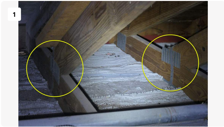
Project: ClubHouse Date: 8/29/2024, 1:29pm Creator: James Stuart
