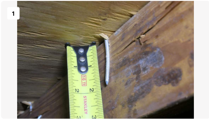
Project: ClubHouse Date: 8/29/2024, 1:27pm Creator: James Stuart
