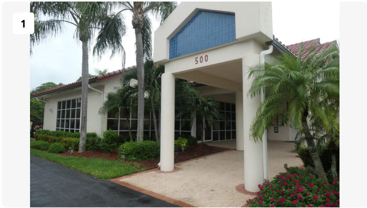
Project: ClubHouse Date: 8/29/2024, 2:06pm Creator: James Stuart
