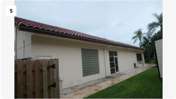
Project: ClubHouse Date: 8/29/2024, 2:09pm Creator: James Stuart
