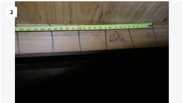
Project: ClubHouse Date: 8/29/2024, 1:28pm Creator: James Stuart
