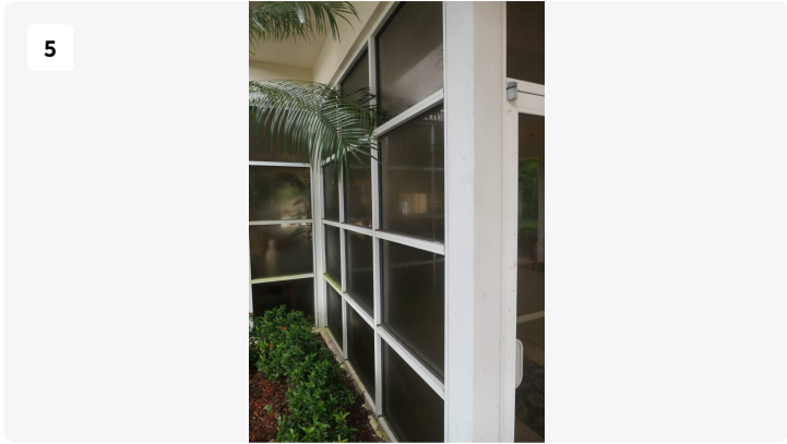
Project: ClubHouse Date: 8/29/2024, 2:07pm Creator: James Stuart
