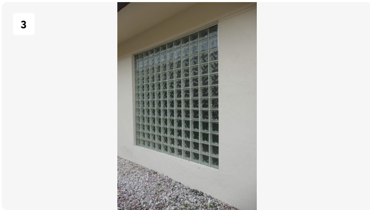
Project: ClubHouse Date: 8/29/2024, 2:09pm Creator: James Stuart
