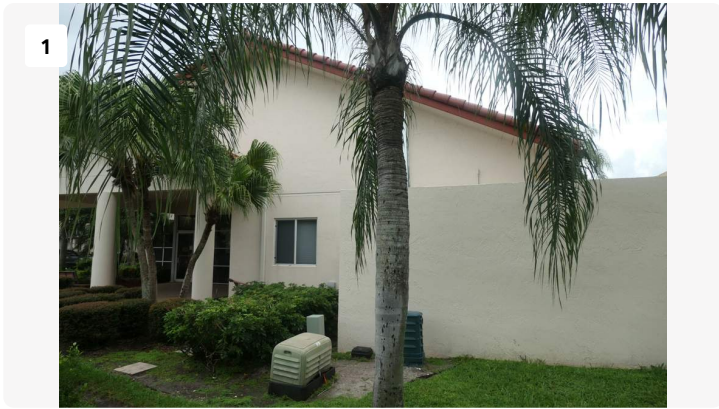
Project: ClubHouse Date: 8/29/2024, 2:11pm Creator: James Stuart
