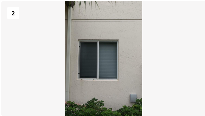
Project: ClubHouse Date: 8/29/2024, 2:12pm Creator: James Stuart
