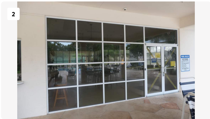
Project: ClubHouse Date: 8/29/2024, 2:08pm Creator: James Stuart
