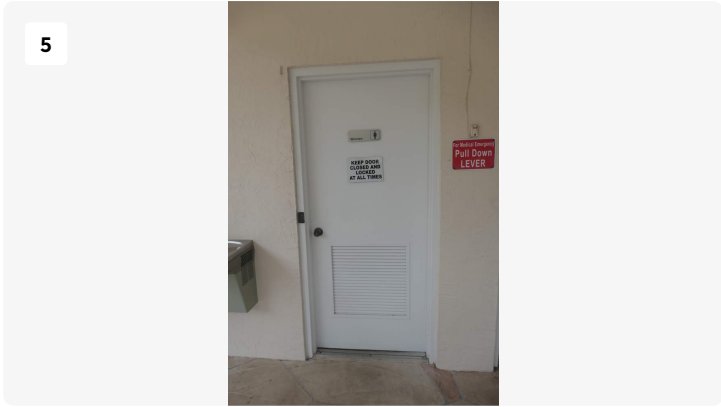
Project: ClubHouse Date: 8/29/2024, 2:09pm Creator: James Stuart
