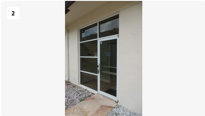
Project: ClubHouse Date: 8/29/2024, 2:09pm Creator: James Stuart
