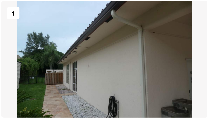
Project: ClubHouse Date: 8/29/2024, 2:09pm Creator: James Stuart
