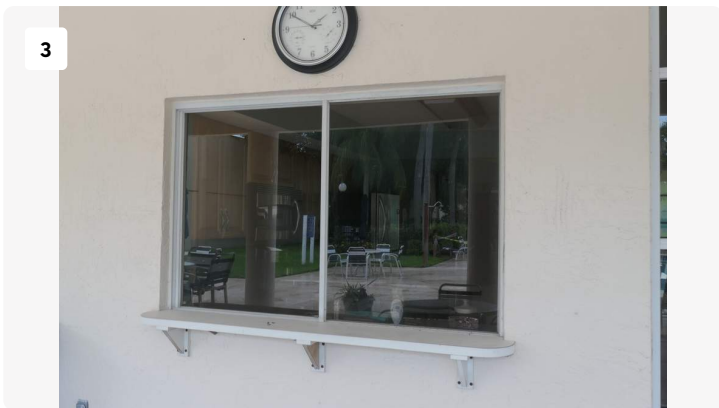
Project: ClubHouse Date: 8/29/2024, 2:08pm Creator: James Stuart
