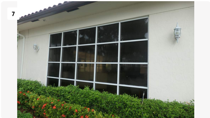
Project: ClubHouse Date: 8/29/2024, 2:07pm Creator: James Stuart
